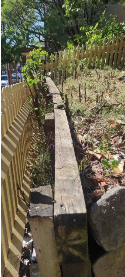
Existing retaining wall
