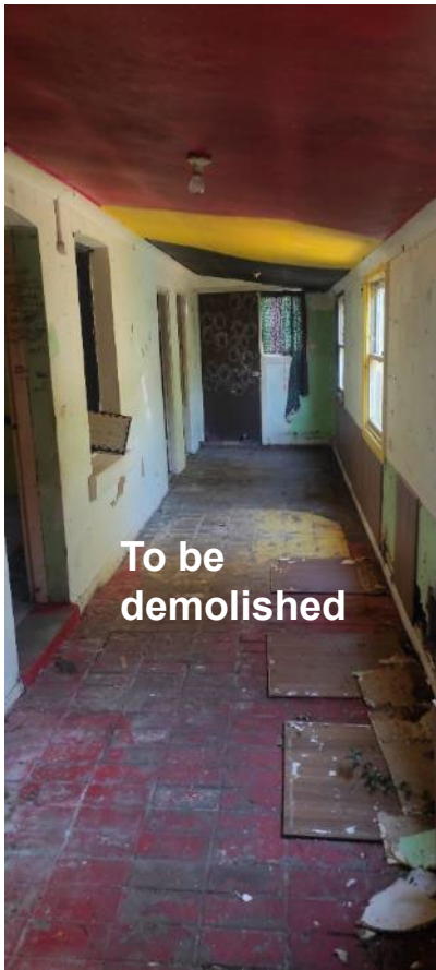
Exiting rear addition
